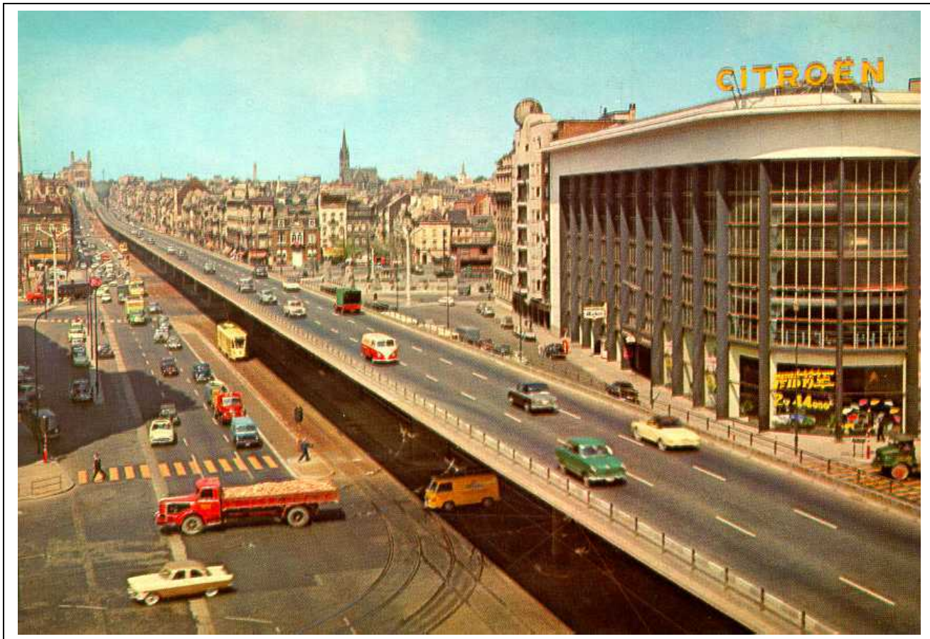
Viaduc Citroën – Note the 'Basiliek van Koekelberg' at the far end of the bridge
